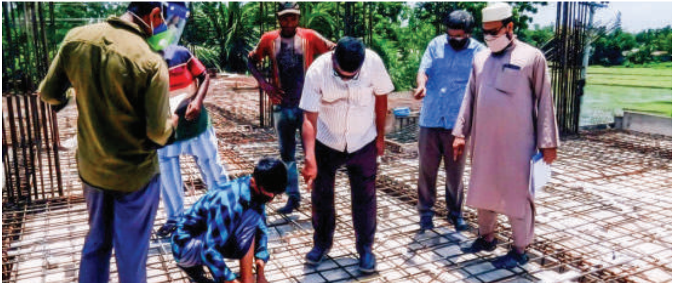
Construction of Dormitory Building
